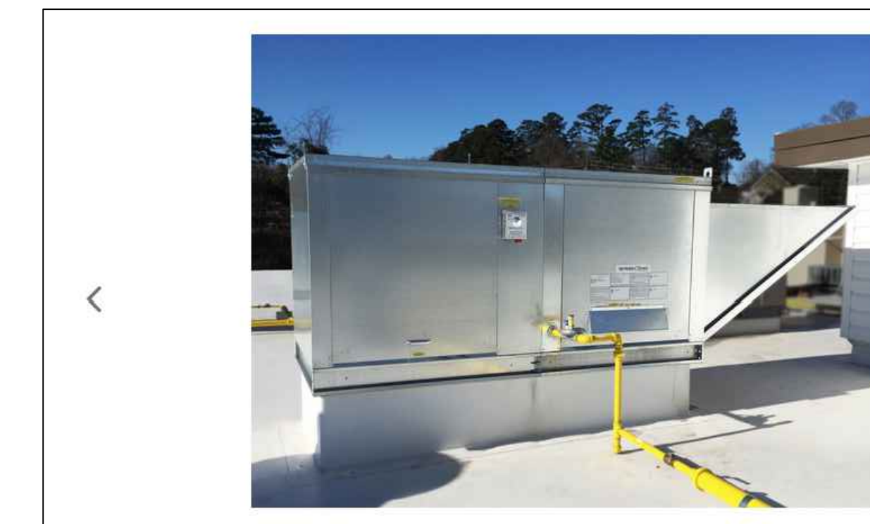
EXIST'G HOT POT AREA MAKE-UP AIR: MUA-1; --5=2880 CFM/208V/20A/3PH
